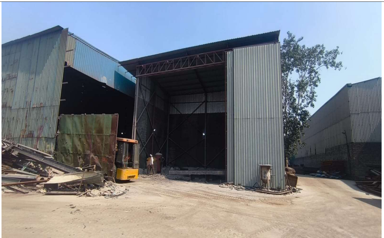
BLASTING & METALISING SHED
