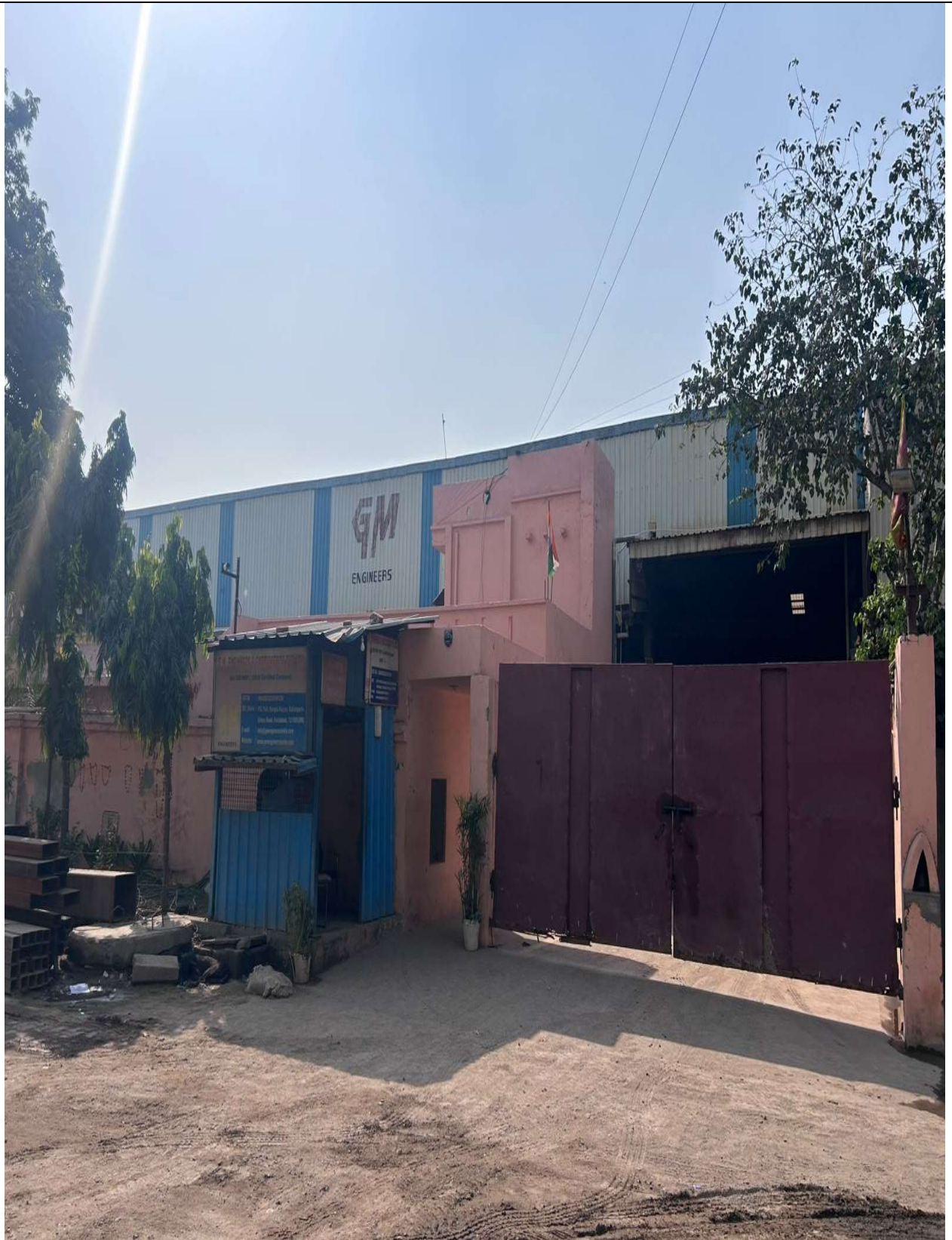
G.M ENGINEERS & FABRICATORS PVT LTD. (FRONT GATE)
